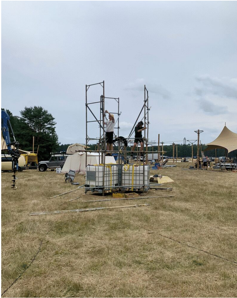
a + r + ibc + scaffolding
